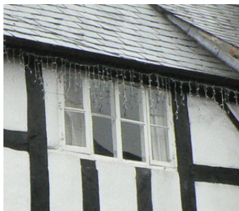
Side-opening Casement in Timber-framed Building
