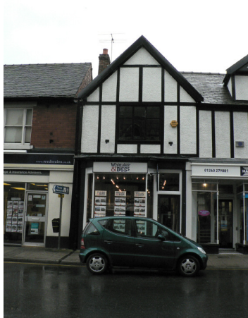
Later Frontage of Number 18 High Street Covering Original Timber Frame
