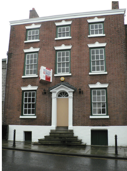
Georgian Building with Six-over-six Sashes without Horns
